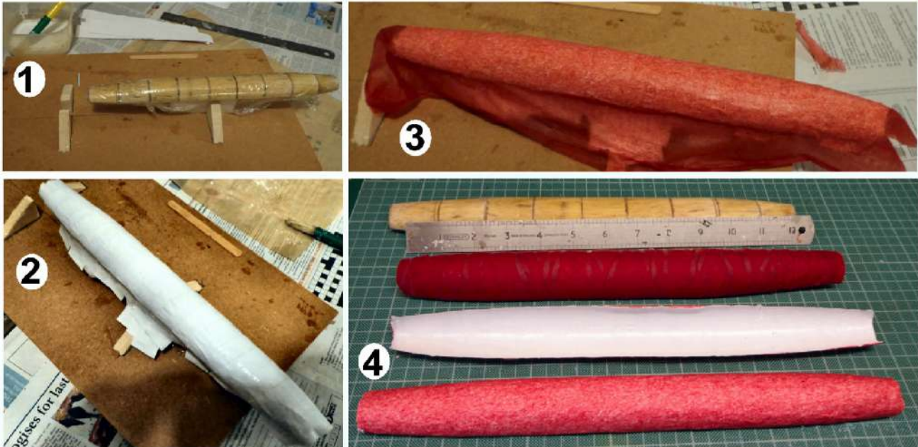
Fig 8:1, the FD 2 mould was mounted and covered in cling film. The diluted PVA glue and 1" wide strips of paper ready for pasting can be seen at the back. 2, three layers were applied diagonally, first one way and then the other. The nose received an extra layer. 3, whilst still wet and looking like the proverbial 'dog's dinner', it was covered with lightweight tissue and dried overnight before taking off the mould and trimming to shape. 4, I made three half fuselage shells, one of 45 gsm paper (front), 60 gsm paper (middle), and, after some cogitation, one of four layers of heavyweight Modelspan tissue (back).
